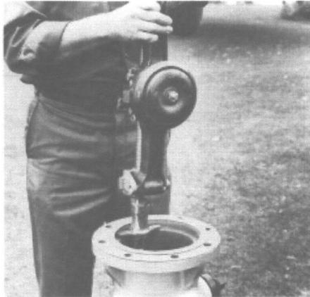
With drain lifter guide 43 in line with the assembly, lower and insert into channel at hydrant bottom, taking care to hold drain valve snugly against back of the hydrant during lowering. If guide 43 is not in line, it will not enter the channel located at the back of the hydrant bottom and the assembly will not slide into proper position.
