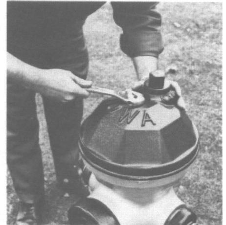
Replace hydrant dome 2, tighten bolt 3.
