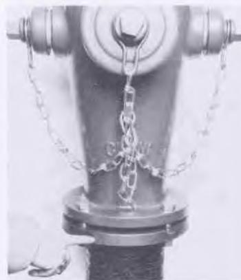
**7** Clean and lubricate gasket recess in nozzle section and position nozzle section on standpipe. Install split break flange (beveled side up). Rotate break flange to line up holes and bolt in place. Torque bolts to 120 ft. lbs. Tighten bolts at overlap of ring first. Uniform space between flanges should be maintained.
