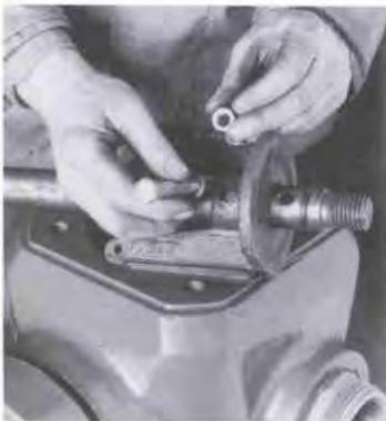
All gaskets and o-rings should be replaced when reassembling hydrant. Any other damaged or worn parts should be replaced as required.
